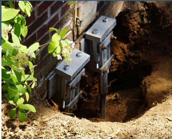
*Foundation problems can be a homeowner's worst nightmare, but with advancements in technology, solutions like helical piles have made foundation repair and stabilization more efficient and effective than ever before.*
