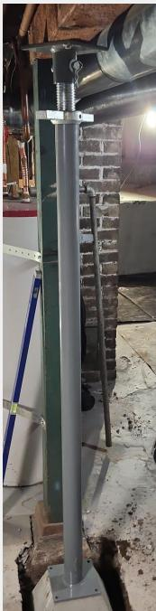
**Adjustable Height:** With the ability to adjust height as needed, these posts offer flexibility in addressing uneven settlement and maintaining a level foundation.
