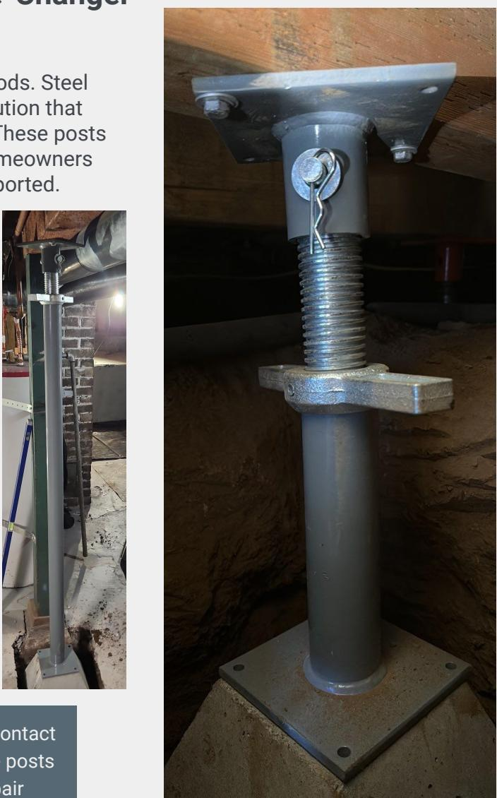
**Reliable Stabilization:** Whether you're dealing with foundation settlement, sagging floors, or uneven surfaces, steel adjustable posts provide reliable stabilization to keep your home structurally sound.
